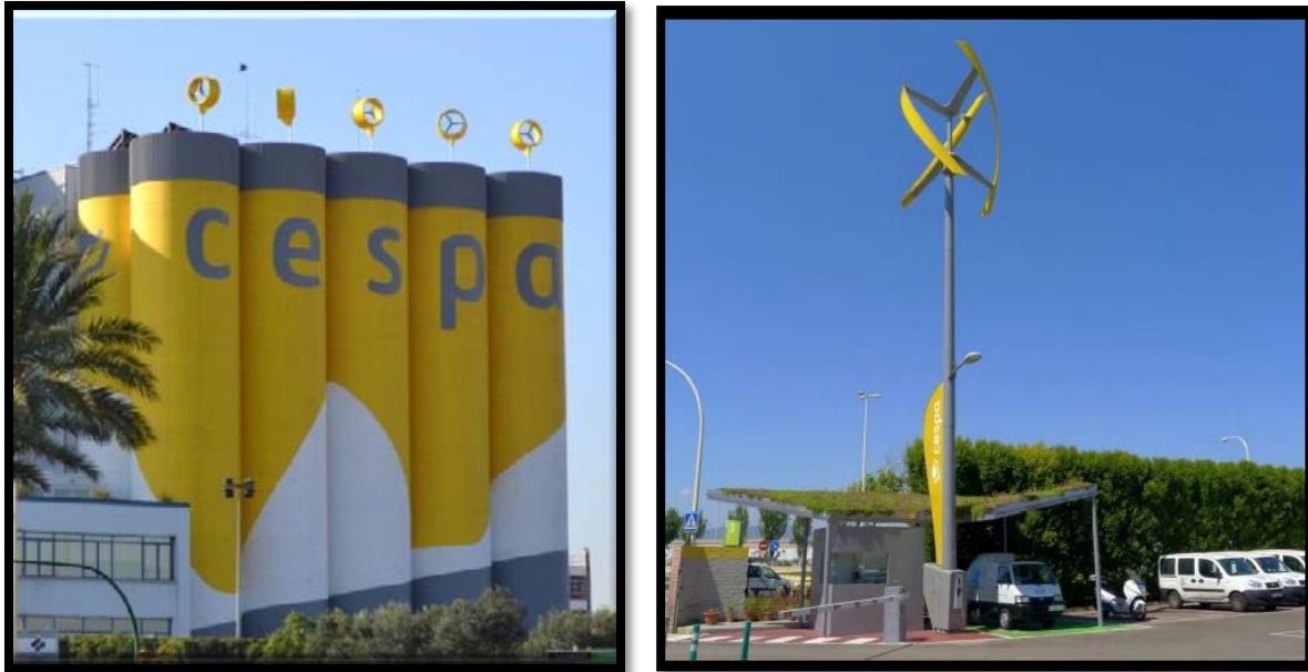
Photo 4: Small-scale wind turbines in Zone Franca, Barcelona's industrial site. On the left, the wind turbine (4kW) charges electric vehicles. Pictures from: CESPA presentation, 2012
